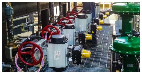
Boiler Blowdown Valves are critical to providing maximum uptime and smooth operations at today's modern power plants. The ability to maintain these valves inline, without cutting them out, saves power plants time and money.
